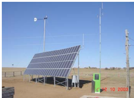
The PV/Wind hybrid system at Naran som, Mongolia
