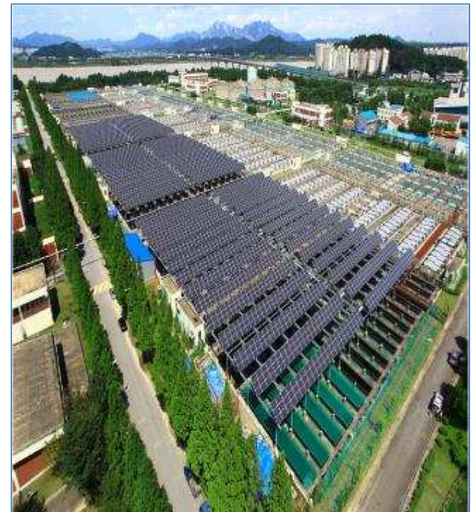
Installation of solar power station at empty site of Arisu Water Purification Center
