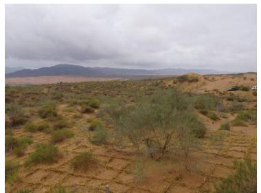
Construction of checkerboard protections to stabilize shifting sand dune. Shrubs are planted within the enclosure of the checkerboard.
